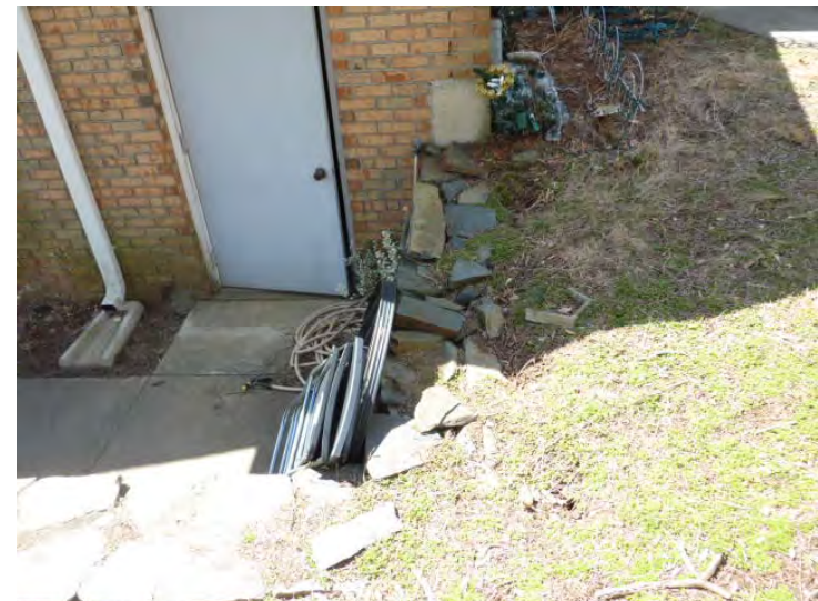
Retaining wall has collapsed and should be replaced. The steel door to mechanical/electrical room does not close or latch and should be replaced.
