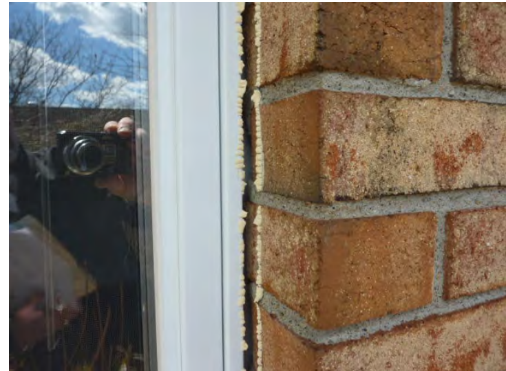
Typical sealant failure at windows, doors, and vinyl siding.
