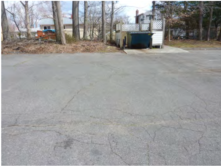
Typical extensive cracking in asphalt paving at parking lots.
