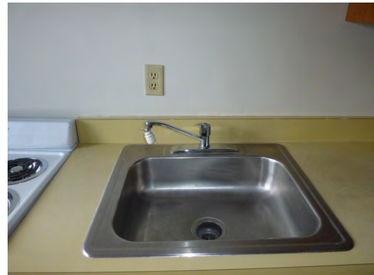
New GFCI outlets should be provided at all kitchen sinks.
