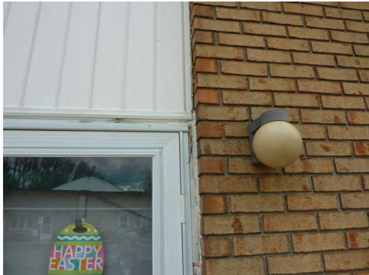
Exterior building light fixtures are worn and should be replaced.
