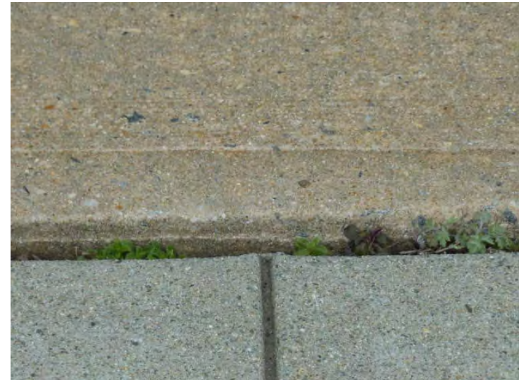
Typical trip hazard at concrete walks and stoops.
