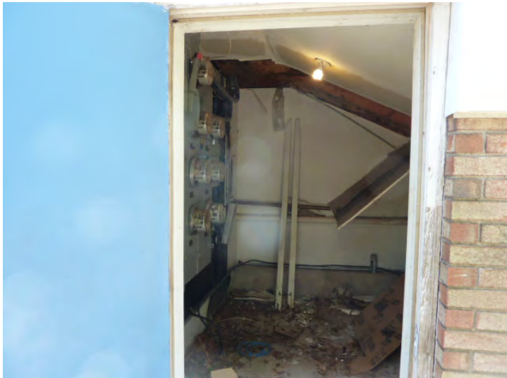
Ceiling has collapsed in mechanical/electrical room.
