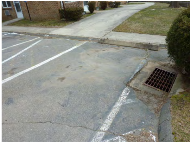
Historic settlement at catch basin and curb, and cracking in asphalt paving.
