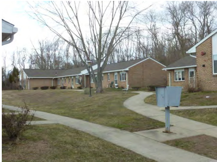
Concrete walks site-wide are in fair condition. Gang mail boxes should be replaced.
