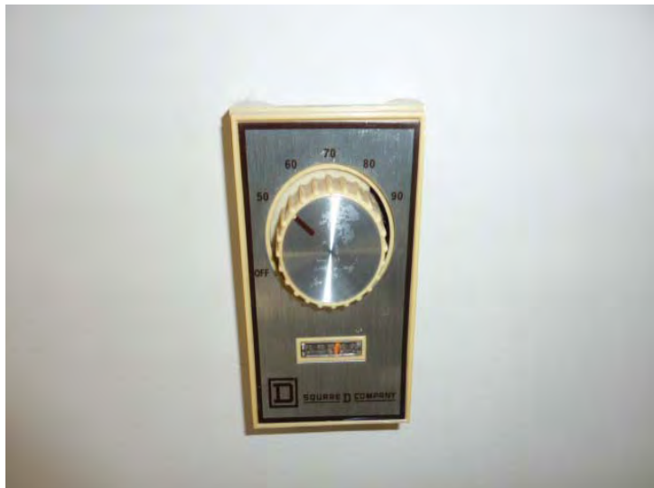
Original thermostats should be replaced.
